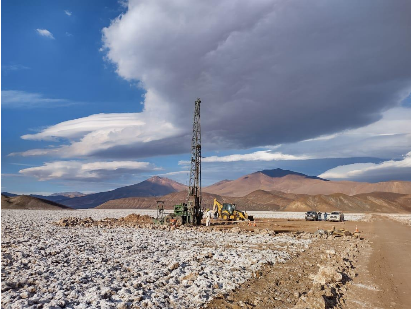
Drill Rig located at drill hole 1 site
